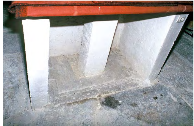
33. Baza oltara ispod konstrukcije novog oltara Base of the old altar beneath the structure of the new altar
