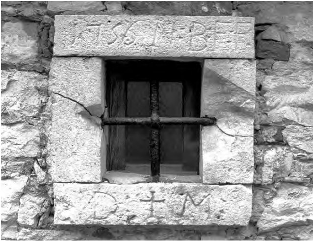
4. Prozor manje sjeverne prigradnje Window in the smaller northern addition
