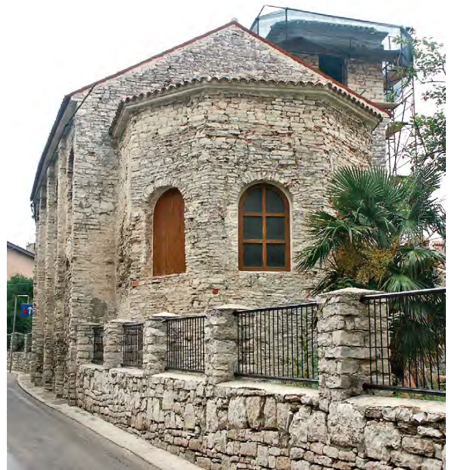
1. Crkva nakon rekonstrukcije pokrova apside i otvaranja prozora (a, b) St Nicholas' after the reconstruction of the apse roof cover and the revealing of windows (a, b)
